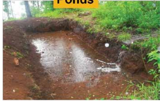
Ground water recharge works on sloping lands to enhance the infiltration of rainwater
