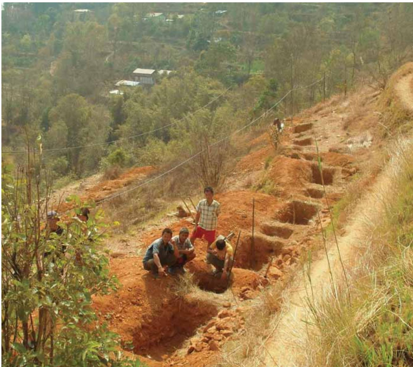
Trenches and pits being dug to capture surface run off on sloping land in the recharge area of a spring to enhance the artificial ground water recharge in order to increase the dry season discharge of the spring
